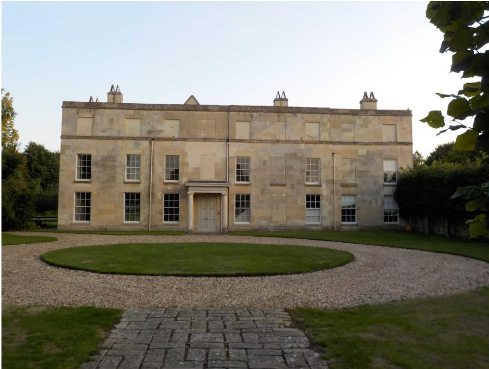
Clatford Hall, Listed No.: 311366
